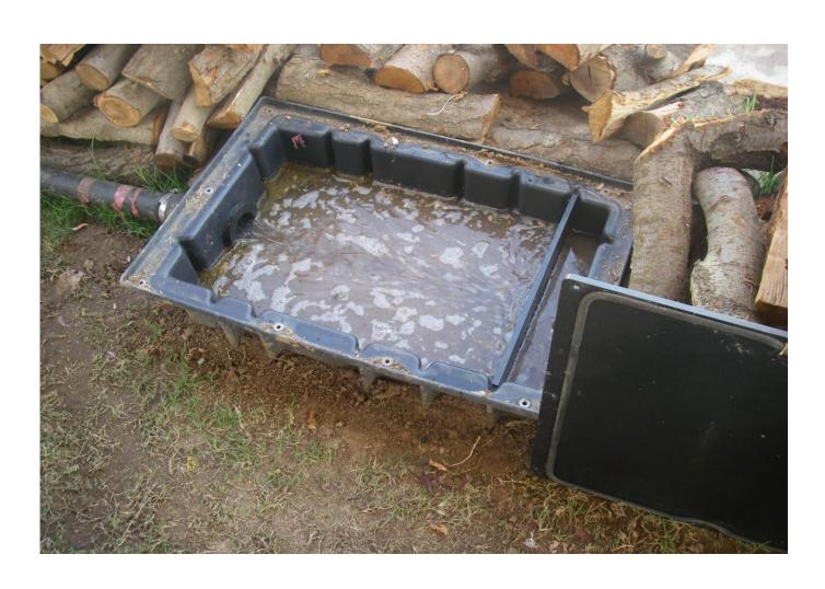
This trap does catch grease and solids if it is properly maintained, meaning staff will not simply lift the baffle wall when it is time to clean and they are in a hurry.
