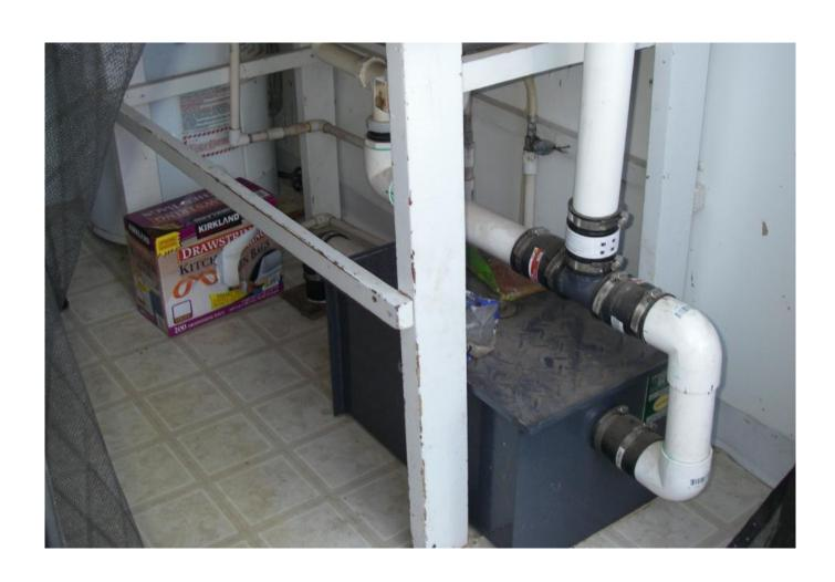
Problem: This pump pushes water to clean out when the float triggers pump. Pump also pushes grease to the clean out. Grease is not being retained.
