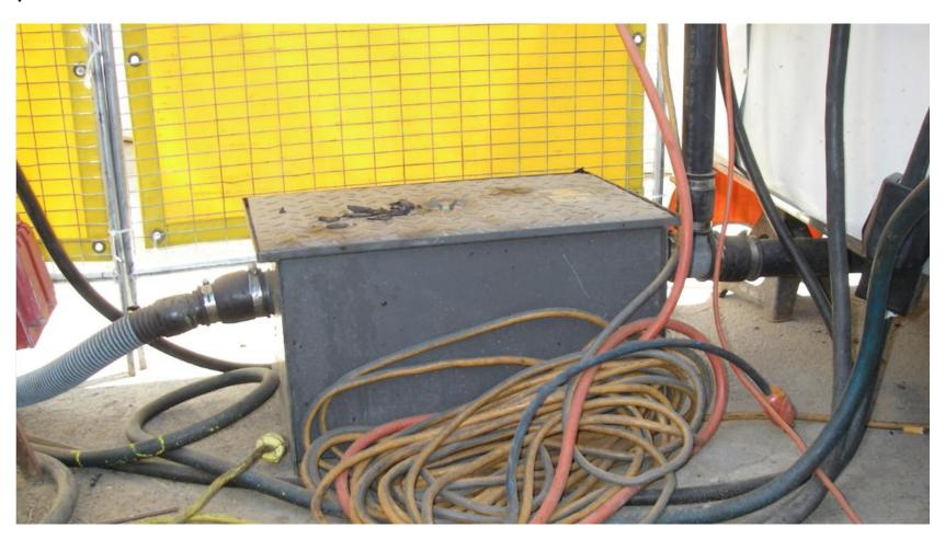
Good: 2" hose; rigid, but smooth, no ripples. Possibly water pump suction hose or hose used in trailer park. Good size trap.
