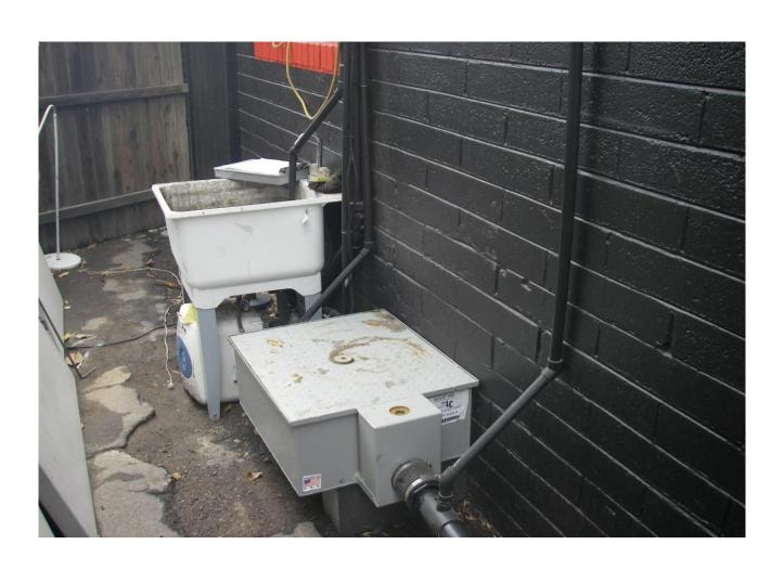
This is a mop sink receiving grey water from a food trailer with a pump. The grey water discharges by gravity to a grease trap with an air vent upstream and downstream of the grease trap.
