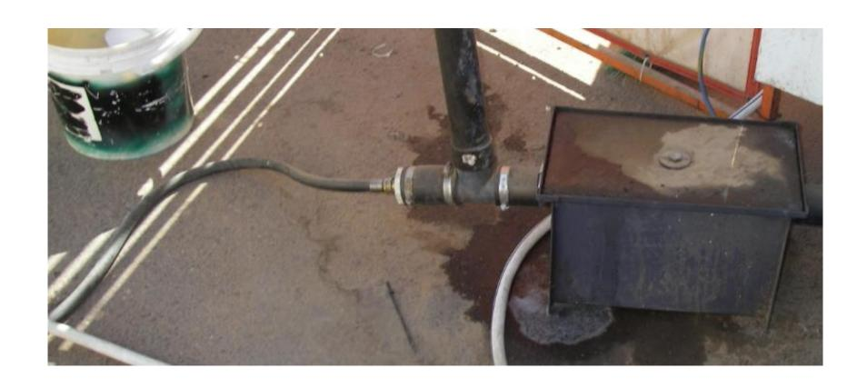
Good: ABS inlet pipe and air vent, good elevation. 2" hose on outlet avoids obstruction. Good sized trap at least 10GPM/20LB.
