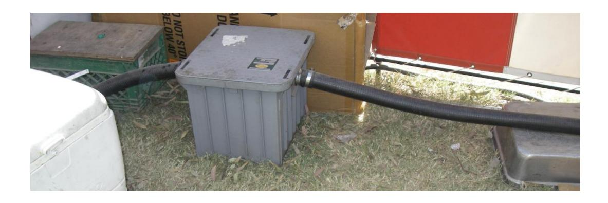
Good: Good elevation on inlet hose. 2" outlet hose avoids obstruction. Good size trap.
