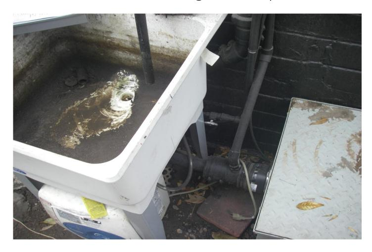
Problem: Not a grease trap. This is a plastic tote with a hole drilled in the side, and the hose sticking out. Vendor replaced this when discovered.
