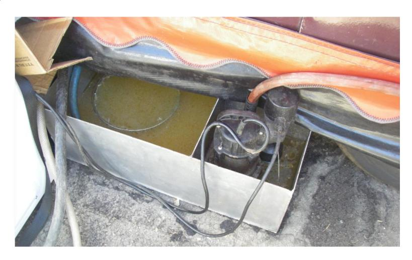
Problem: Pump in trailer forces water into trap, disrupting grease and preventing it from separating in trap. Pump in trap sends grease along with water to clean out. Grease is not being retained.
