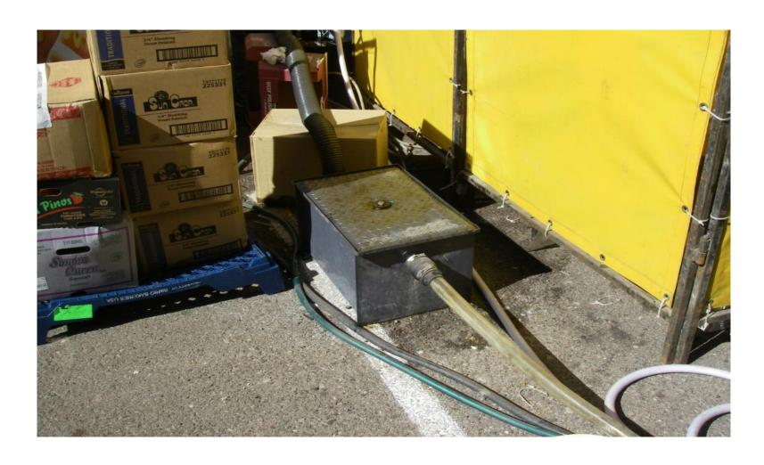
Very good: PVC for inlet pipe and air vent. PVC outlet pipe, all the way to cleanout. Good size trap.
