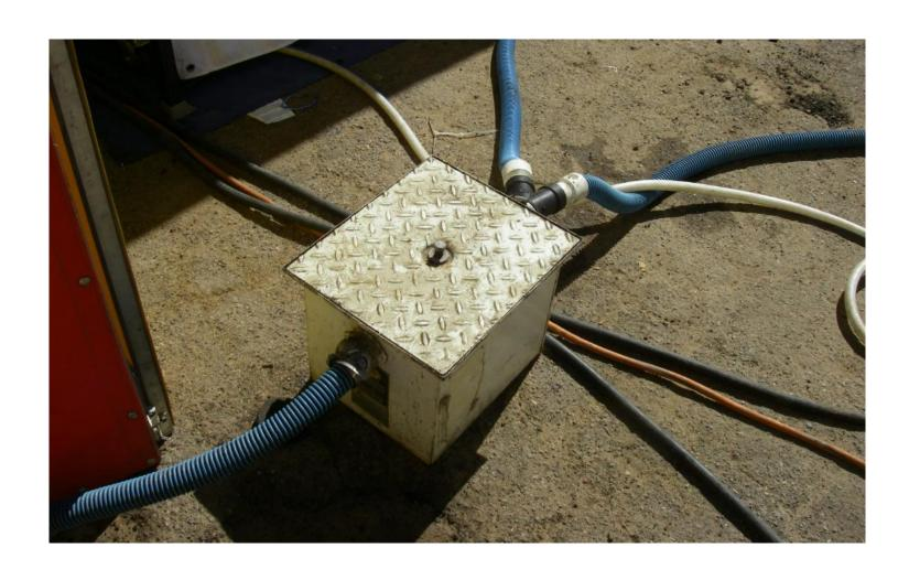
Problem: Outlet hose is only a 5/8" garden hose. This will cause an obstruction in trap or before trap, and could cause a spill. The downstream air vent is a great idea but not mandatory.
