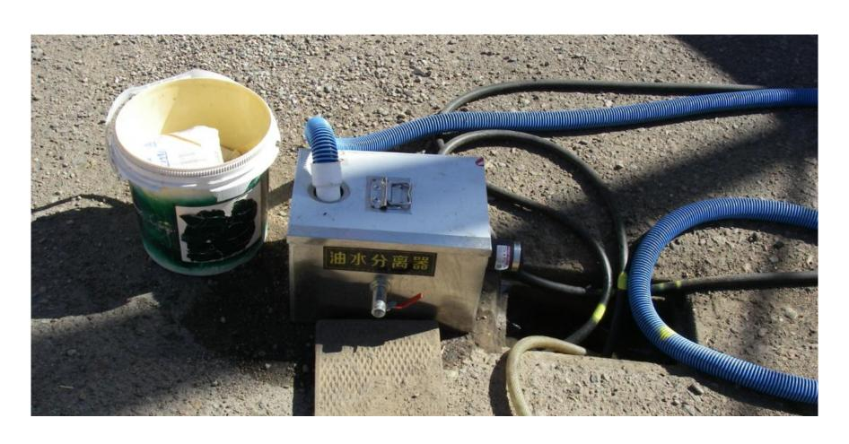
Problem: Inlet hose is below the level of grease trap inlet. This will create an obstruction and water will not enter trap with proper flow.
